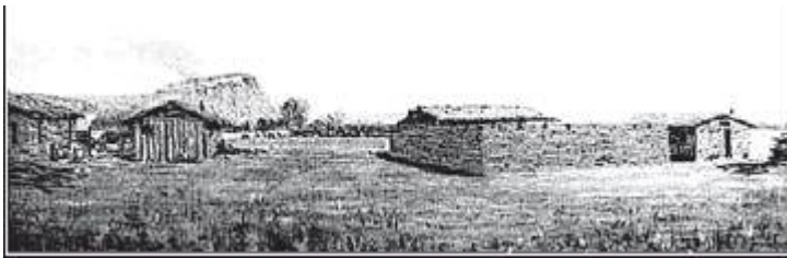
Adobe walls. [PROVIDED BY CHUCK LANEHART]
